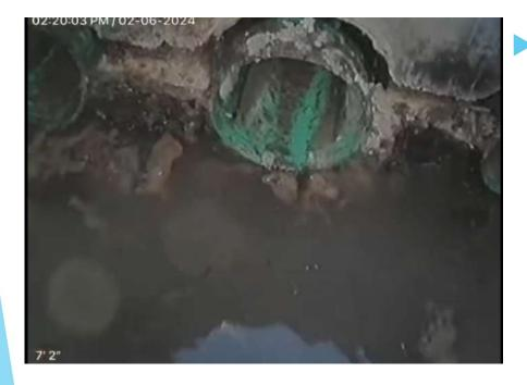
Distribution box is not water-tight, some off the effluent may not get secondary treatment
