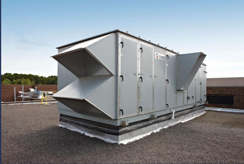
TOP LEFT: AIR HANDLER / PACKAGE UNIT INSTALLED AT COLLEGE
